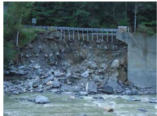
Fig. 3.2.10 Cold River Bridge Florida/Savoy
