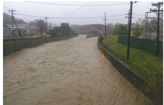
Fig. 3.2.12. Flood Control Chutes in North Adams
