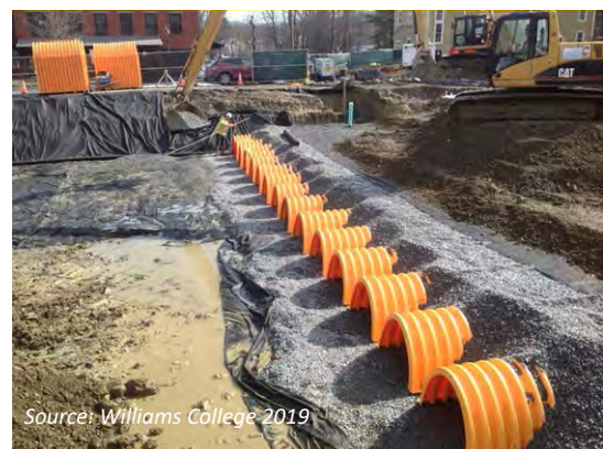
Fig. 3.2.14. Parking Lot Infiltration System being Installed
