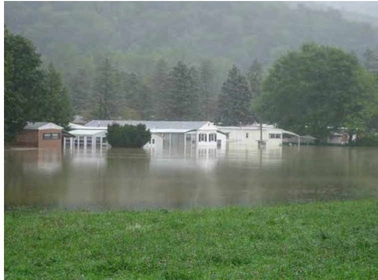
Fig. 3.2.9. Flooding of The Spruces Aug. 28, 2011; water is approximately 5' in depth
