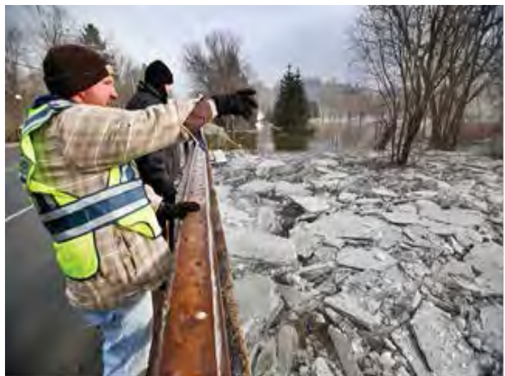
Fig. 3.2.9. Ice Jam on Housatonic River, Rt. 7 Stockbridge Jan. 2018
