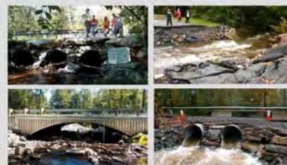
Clockwise from top left: First replacement culvert (2006), culvert failure due to Tropical Storm Irene (2011), temporary temporary replacement culvert (2012), replacement bridge (2016).
