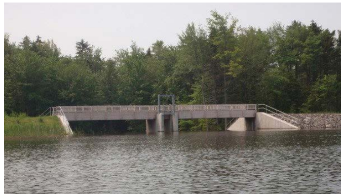
Fig. 3.15. Lake Ashmere Dam spillway
