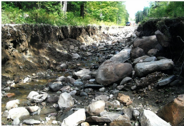
Figs. 3.10-3.12. Hickingbotham Rd. after T.S. Irene 2011. Top Left: looking up washed out section of road; note truck at top for scale. Top Right: Looking down that same section. Bottom: Washed out road underlayers.
