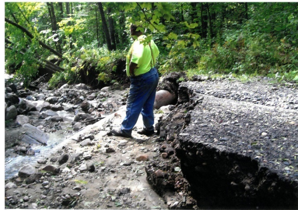
Figs. 3.10-3.12. Hickingbotham Rd. after T.S. Irene 2011. Top Left: looking up washed out section of road; note truck at top for scale. Top Right: Looking down that same section. Bottom: Washed out road underlayers.
