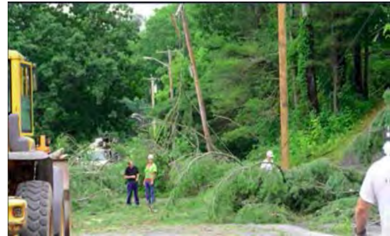
Fig. 3.24. Microburst damage in Cheshire, 7-18-16
