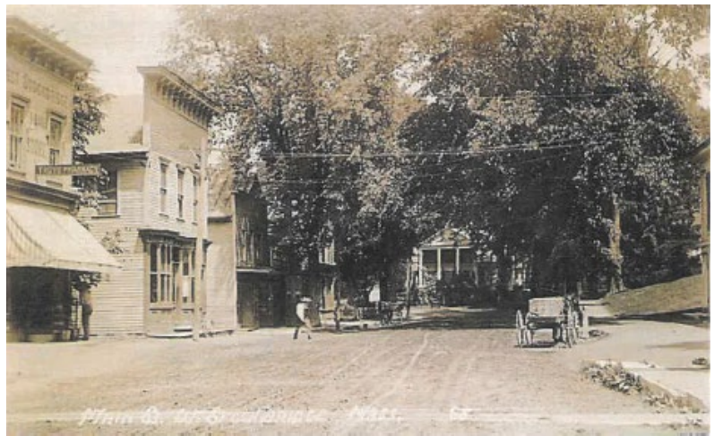
Fig. 4.5. View of the North section of Main Street
