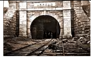
Western portal of Hoosac Tunnel
