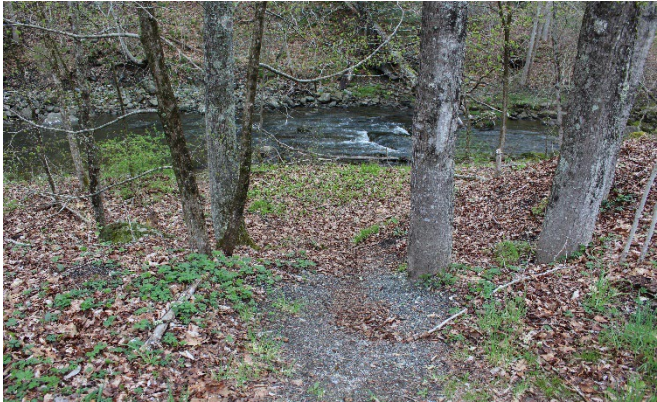
A steep slope down the riverbank limits the town’s ability to further the develop the property in an ADA compliant manner.
