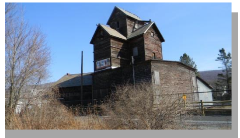
The former Hoosac Valley Coal and Grain site along the Ashuwillticook Rail Trail. The grain elevator is shown.
