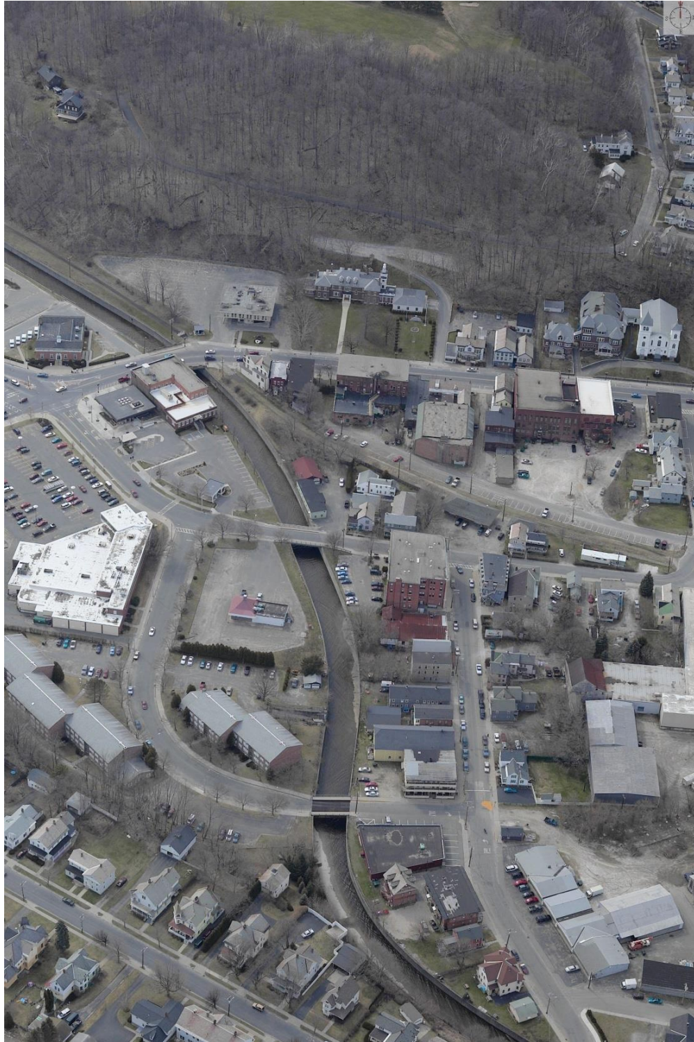
Figure 6: Aerial View of the Flood Chutes through Downtown Adams
