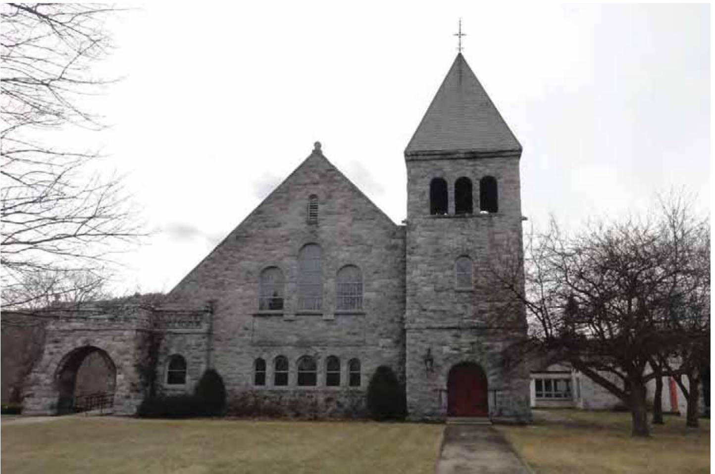
Figure 9-5. Historic First Congregational Church
