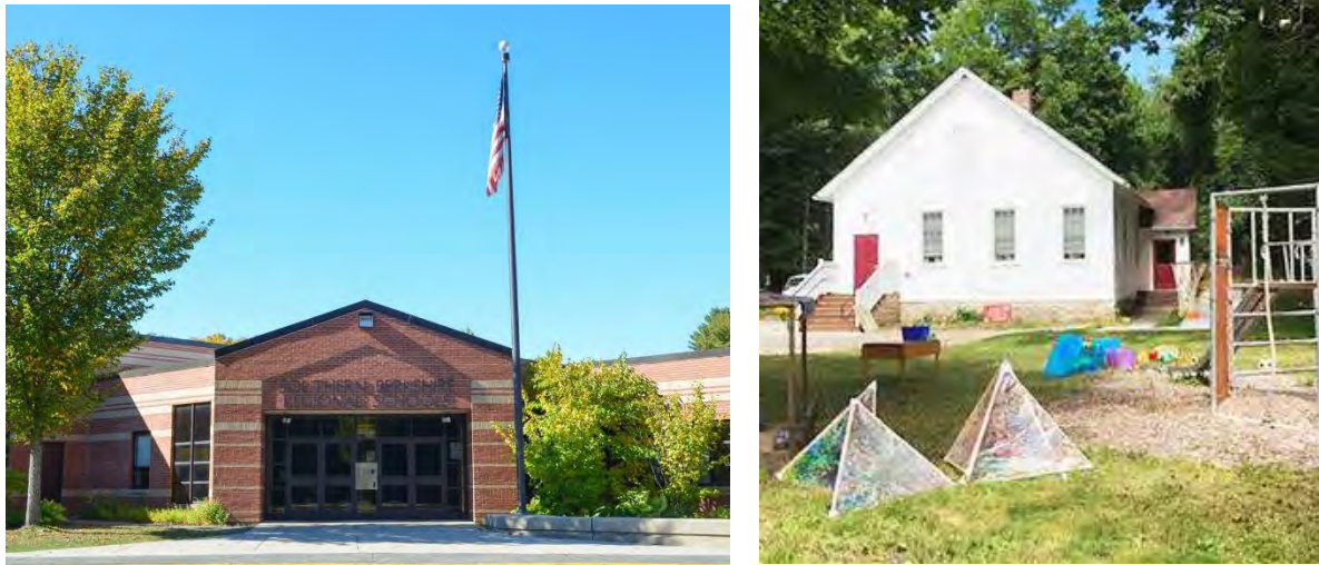
Figure 3-1. Southern Berkshire Regional School District; South Egremont Elementary School (SBRSD, 2021)
