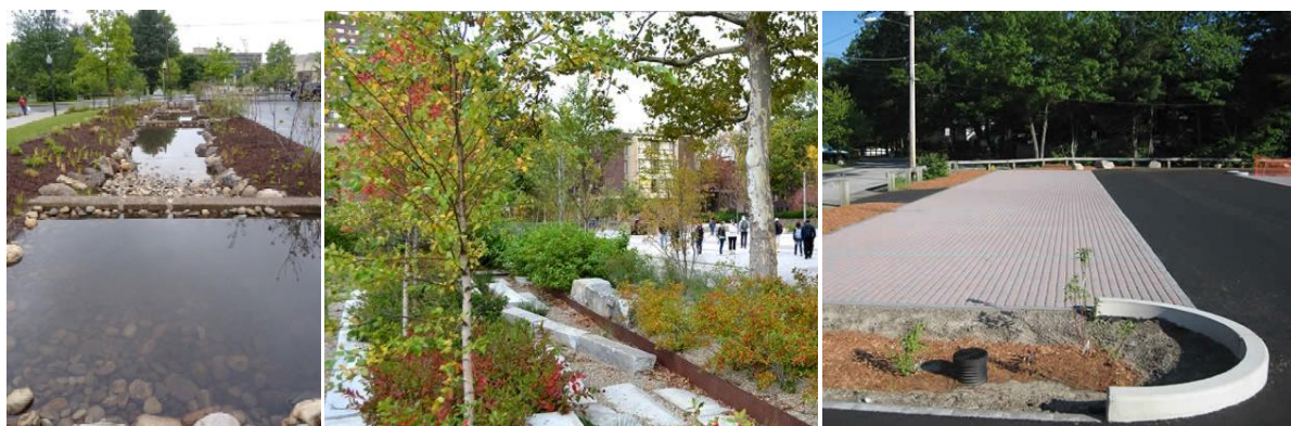
Two examples of green infrastructure at UMass-Amherst: On the left, a bioretention swale catches storm water and slows it down, allowing it to cool and percolate into the ground instead of flowing quickly, full of sediment, into the Mill River and its wetlands. On the right, a rain garden on the UMass-Amherst campus provides a beautiful space to relax while providing water slowing and filtering services. A parking lot in Wilmington (MA) uses permeable pavement and a swale to reduce water runoff at a lake-side recreation area.
