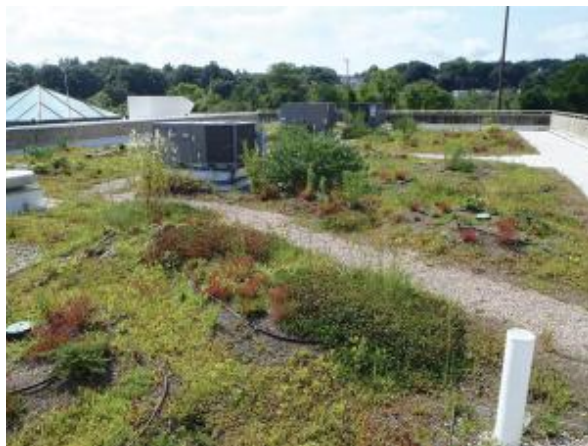
Two examples of green roofs in Massachusetts communities: An 'intensive' roof growing flowering plants and shrubs, including blueberry plants, on the right, at the Lowell Regional Wastewater Utility. An 'extensive' system, with different varieties of low growing, drought-tolerant plants, on the left, at a senior housing complex in Ipswich.
