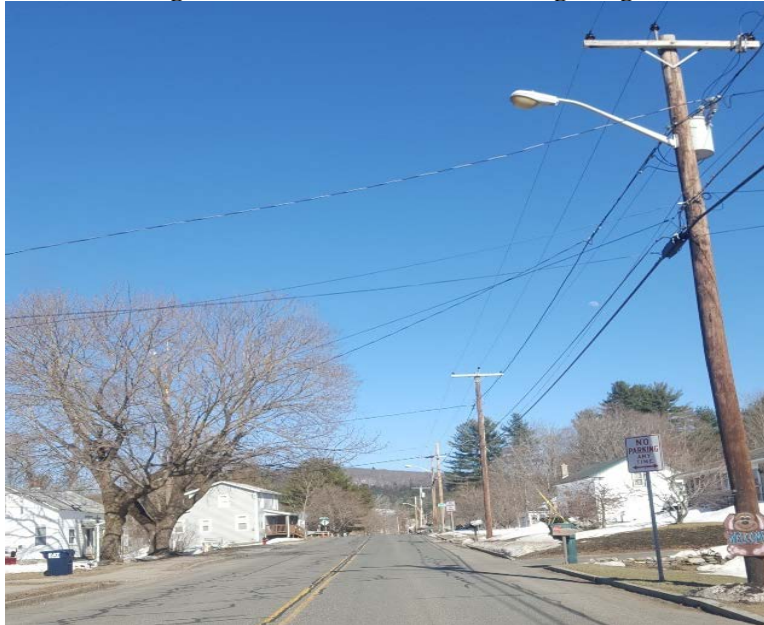
Figure 4.3 Main Street – Street Lighting
