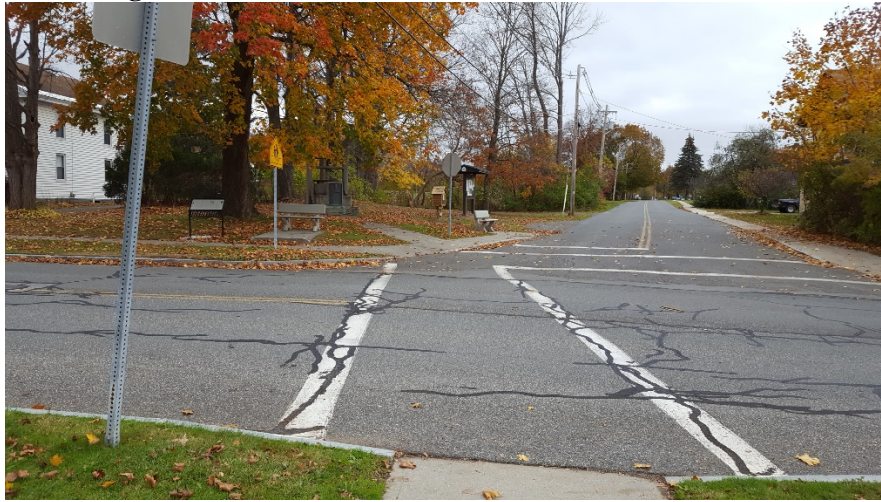
Figure 4.4 Intersection of Church Street & School Street
