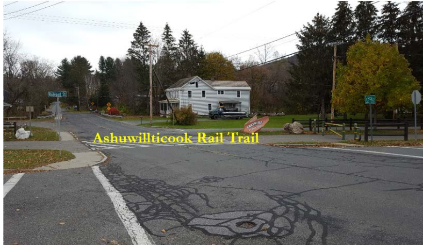
Figure 4.1 Ashuwillticook Rail Trail Crossing on Church Street
