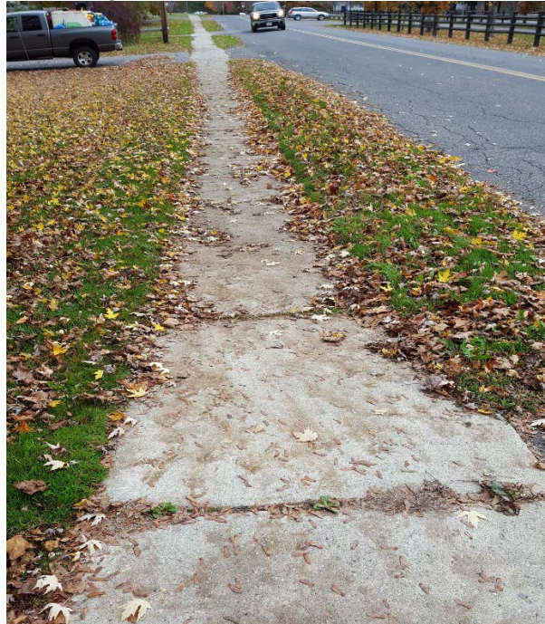
Figure 4.7 Railroad Street Sidewalk
