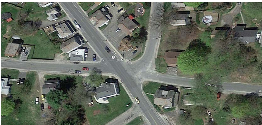
Figure 33. Intersection of East Main St. and Route 2
