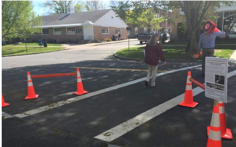
Figure 5.2 One of Two Temporary Curb Extensions Installed on Main Street 2017
