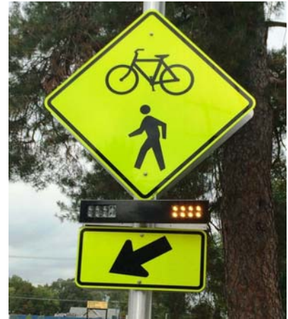
Figure 5.8 Rapid Rectangular Flashing Beacon
