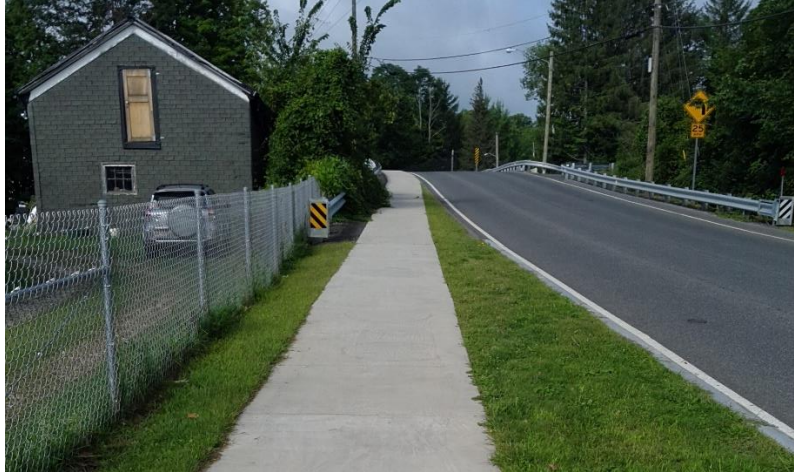
Figure 12. Sidewalk on Bridge Street in Excellent Condition
