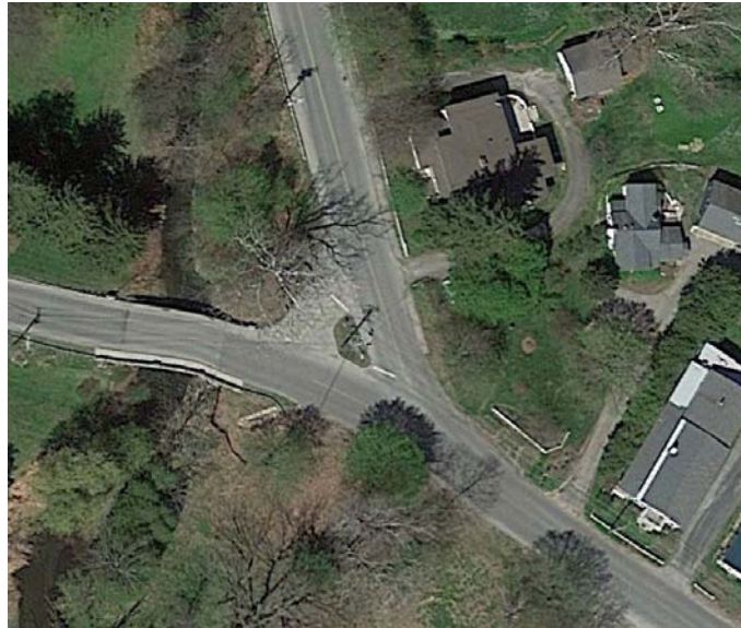
Figure 15: Intersection of Buttonball Lane and Sheffield Road
