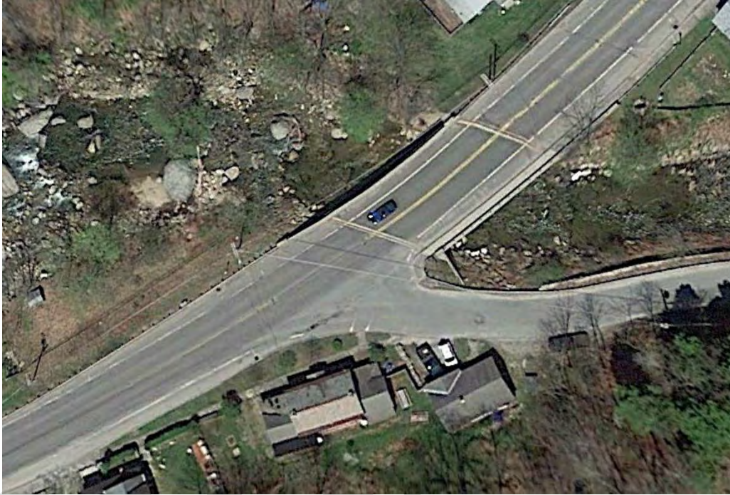
Figure 17. Intersection of East Rd. and Route 8.
