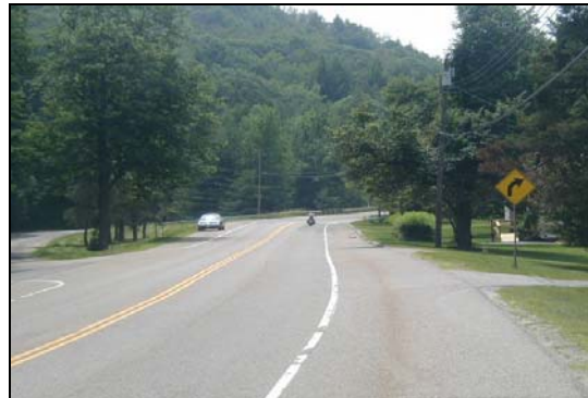
d) Roys and Greylock intersections, looking south
