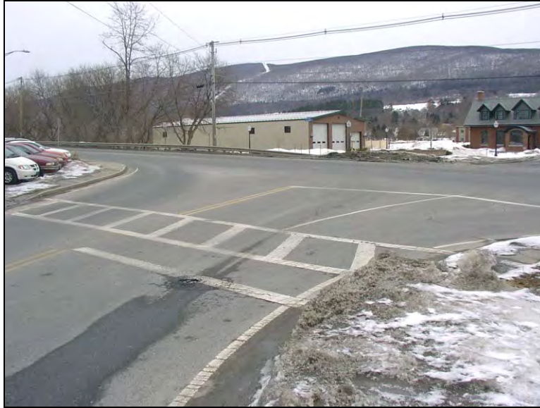
Figure 6: Stop lines and pedestrian crossing on Friend Street
