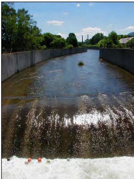
Figure 5. The concreted Hoosic River channel keeps flood waters out of downtown Adams.
