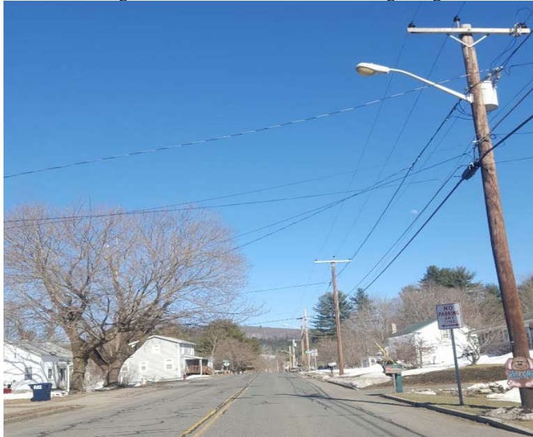
Figure 4.3 Main Street – Street Lighting
