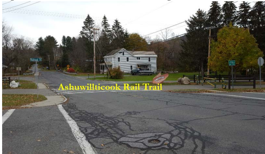
Figure 4.1 Ashuwillticook Rail Trail Crossing on Church Street
