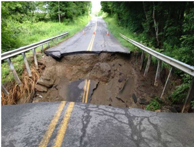
Image 3a and Image 3b Heavy rain damaged and closed Windsor Road June 2014
