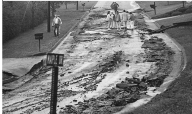
Image 4 Savoy Road washout 1988
